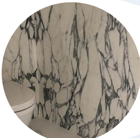
F ull-height marble slab bath walls (181 Fremont)
