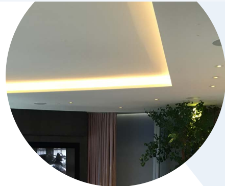
R ecessed cove soffit lighting (181 Fremont)
